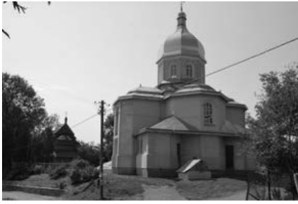
Figure 6 Wooden Church of Assumption of Blessed Virgin Mary (1604) and the new church construction Klits'ko village (August,
