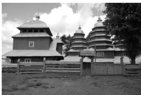
Figure 4 Wooden Church of St. Dmytro (1838), Matkiv village (July, 2015)
